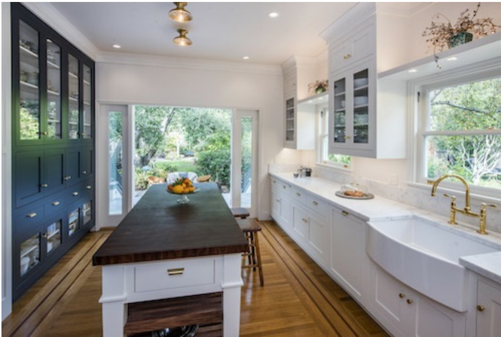
RECO installed uplights and undercounter strips that help save energy
